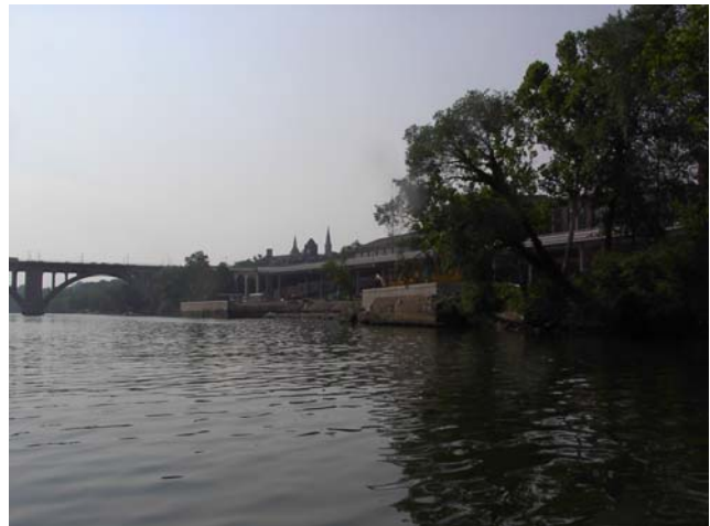
Photo 7-3. Shoreline armoring in Georgetown, with Key Bridge in the Background. June 2007
