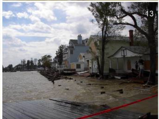
Photos 9–15. Chesapeake Beach and North Beach the Day after Isabel. The beach at Chesapeake Beach has almost all been replaced by stone revetment, which protects against erosion but not high water (9). The new condominiums have first floors elevated to the base flood elevation, but owners suffered substantial uninsured losses because most had improved the floor below the first floor. As late as 2:00 p.m., the Bay was still over the road between Chesapeake Beach and North Beach (10), and several feet deep throughout low-lying areas of North Beach (11–12). The most severe damage occurred along the boardwalk section of Atlantic Avenue (13), although flooding was also severe along the avenue's paved portion (14–15).
